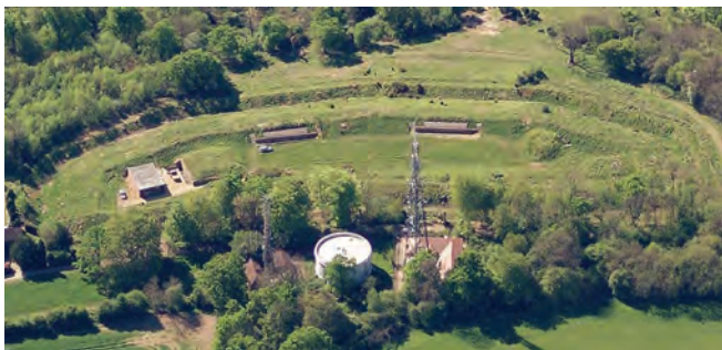
Reigate Fort – the buildings are from left to right: Tool store, Underground Magazine, Casemate, Casemates (initially used for storing entrenching tools)
